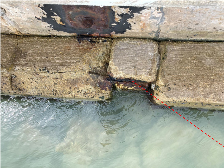
Photo #4- View of Spalling Stress Beam.
