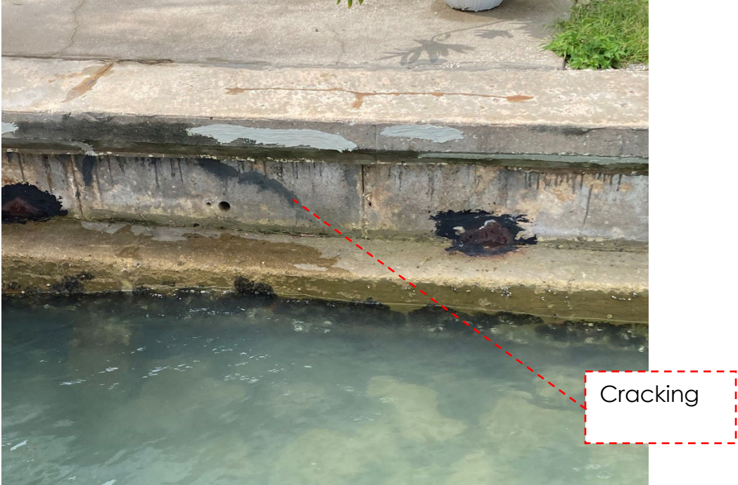
Photo #10- View of Cracking in Top of Cap.
