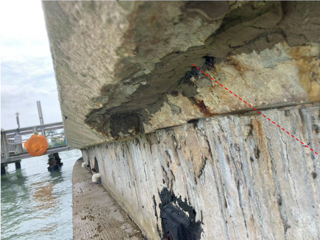
Photo #6- View of Spalling of Bottom Front Face of Cap.
