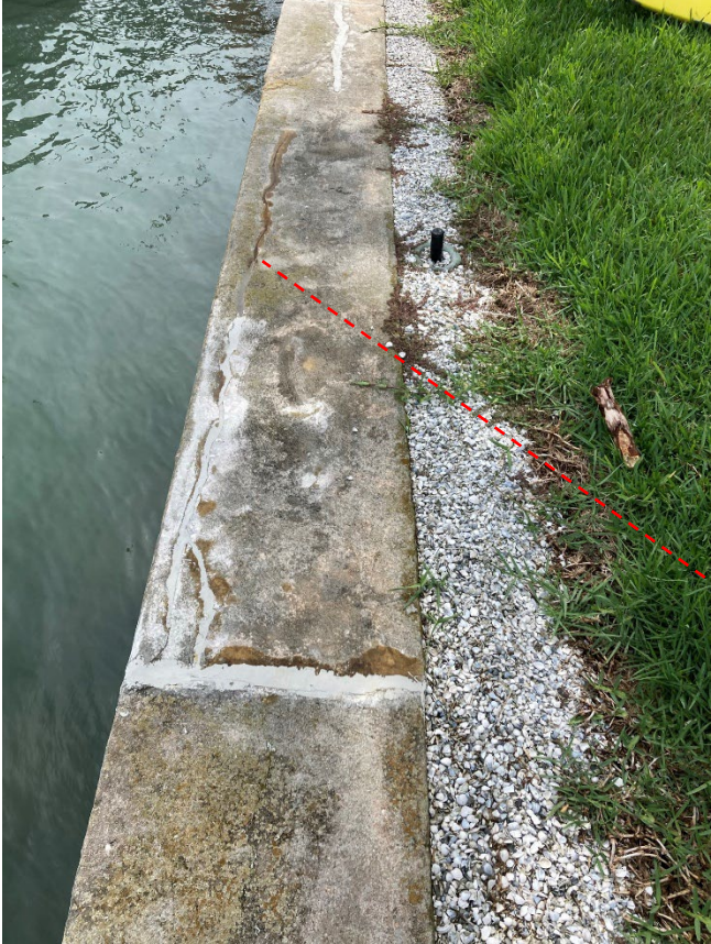
Photo #6- View of Spalling of Bottom Front Face of Cap.
