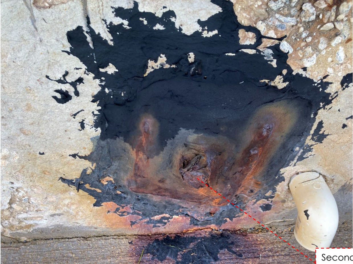
Photo #4- View of Spalling Stress Beam.
