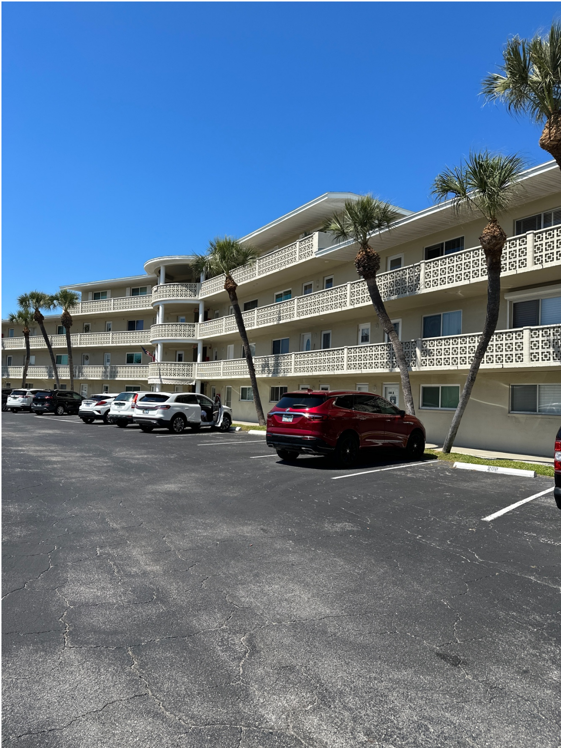
Front (South) Elevation of Building
