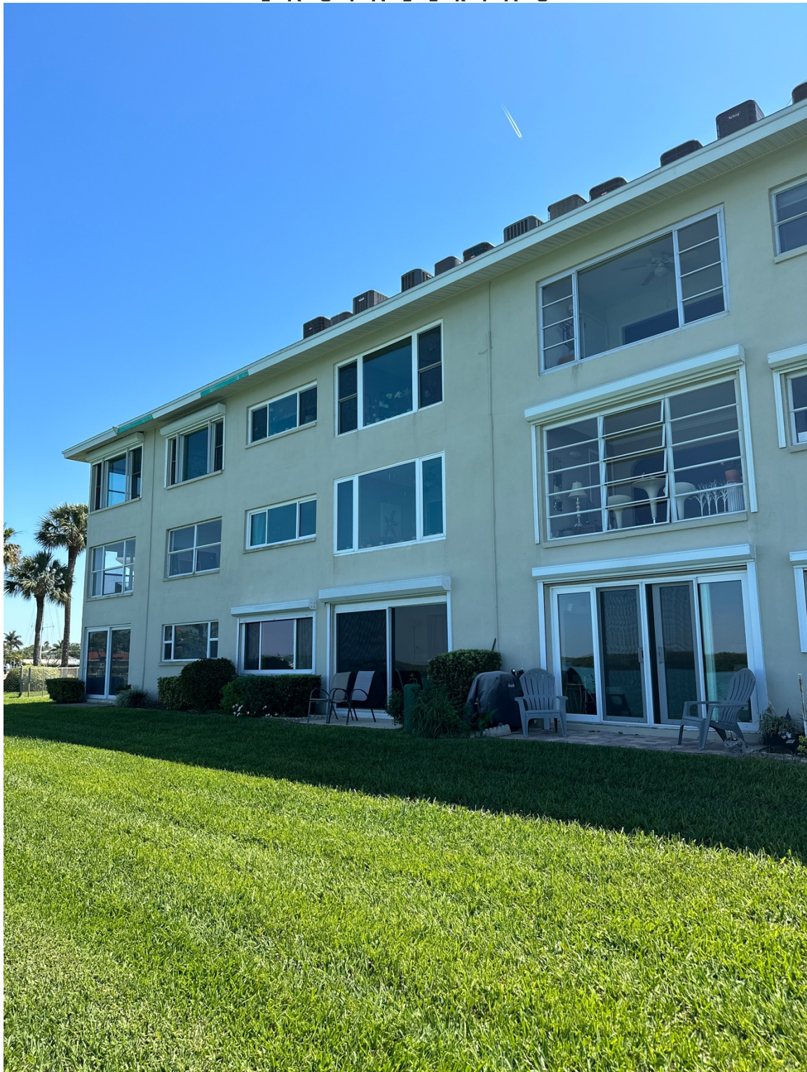
Rear (North) Elevation of Building
