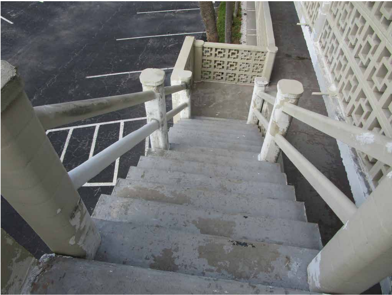
Capri Isle Garden Apartments No. 2. Typical exterior stairs.
