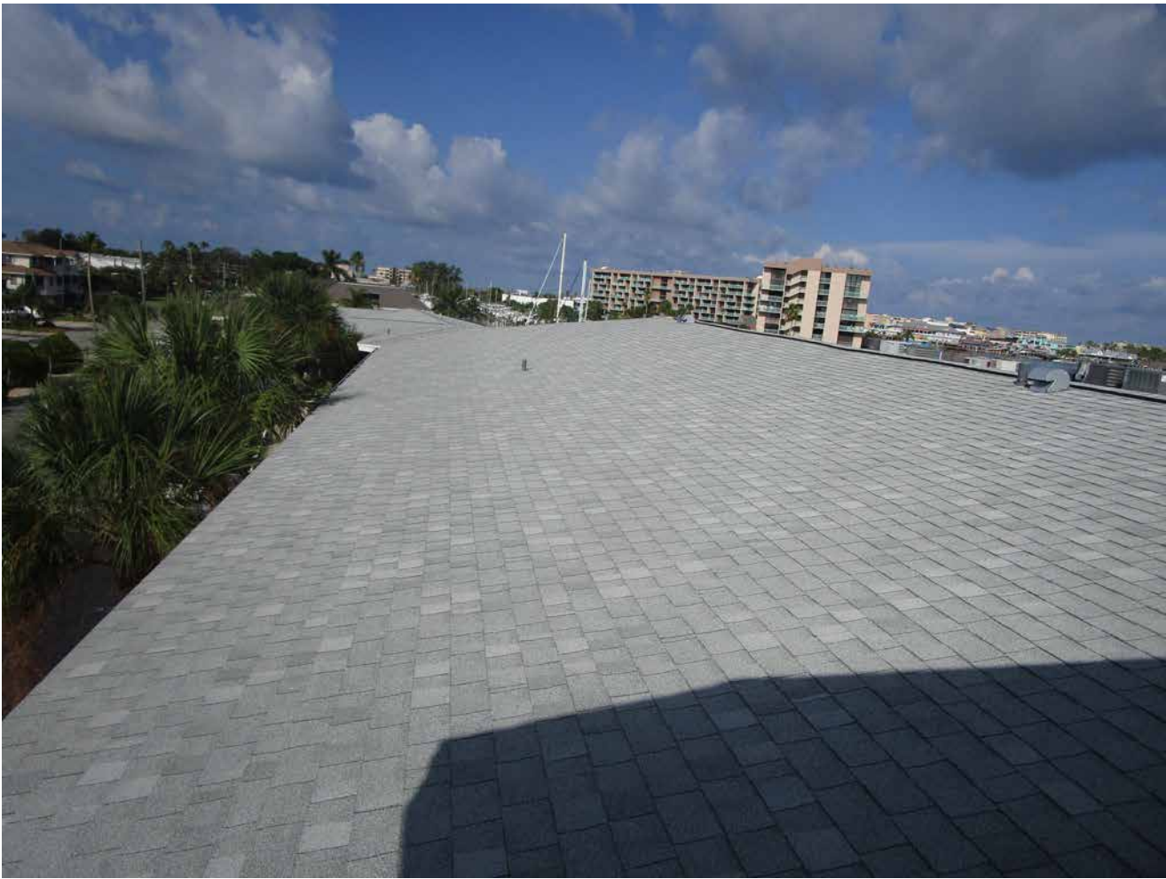
Capri Isle Garden Apartments No. 2 , typical roof area.
