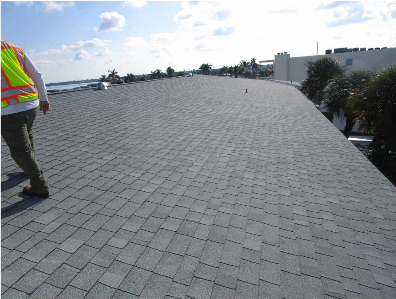
Capri Isle Garden Apartments No. 2. Roof shingles are in good condition.
