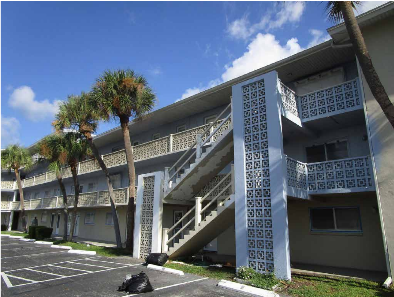
Capri Isle Garden Apartments No. 2. Front (South) elevation.
