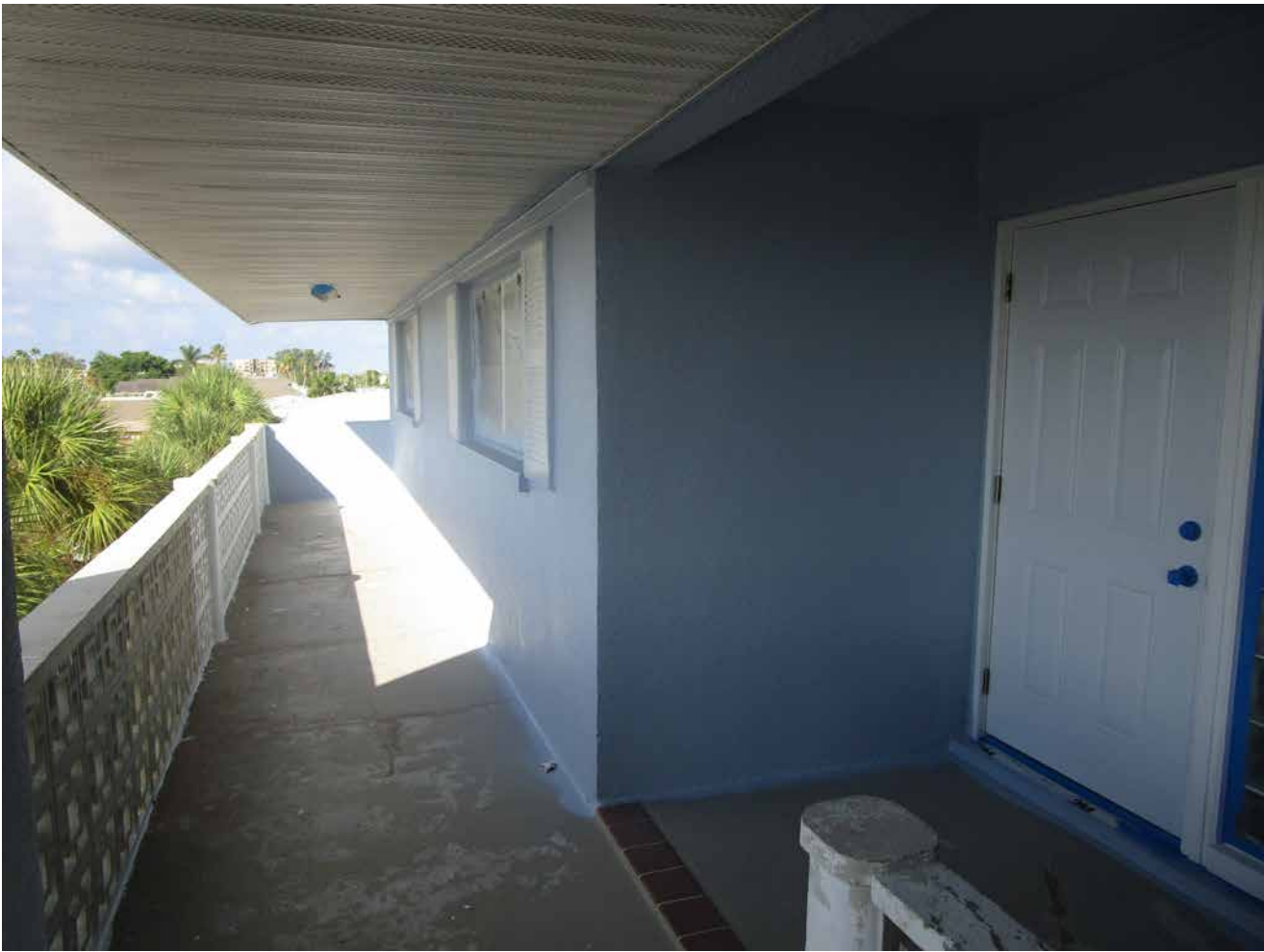
Capri Isle Garden Apartments No. 2 , typical walkway area.
