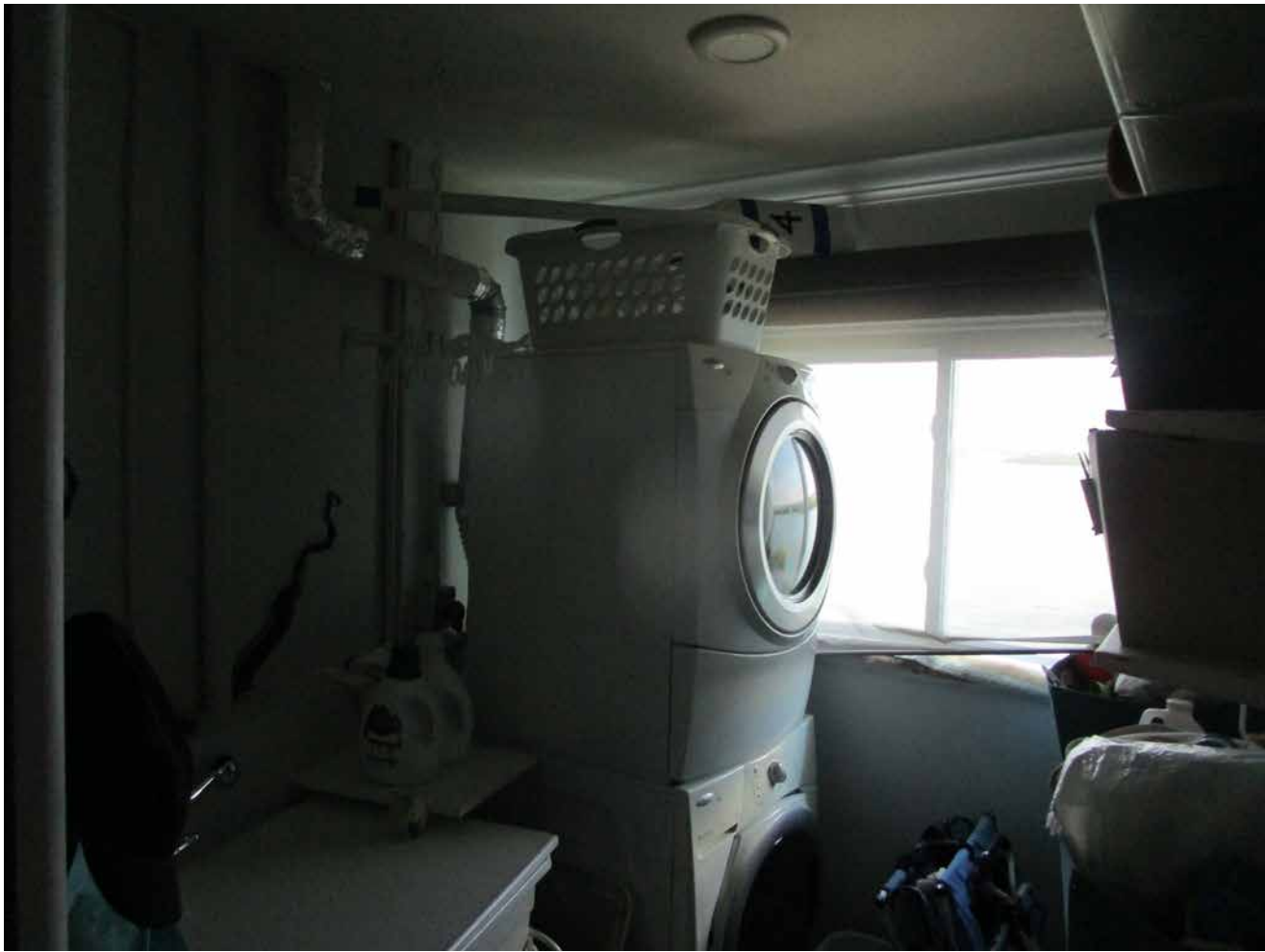
Capri Isle Garden Apartments No. 2. Unit 401. Minor cracking in interior ceilings observed, which is typical for this construction. This is not a structural issue and no action is required.
