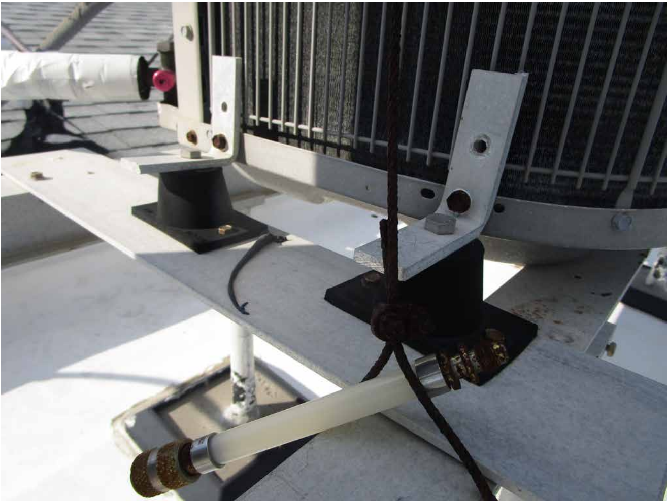
Capri Isle Garden Apartments No. 2.
