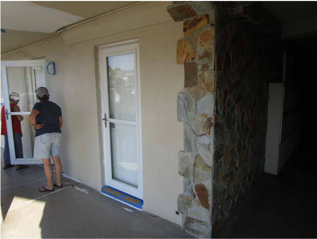
Capri Isle Garden Apartments No. 2. ground floor walkway.
