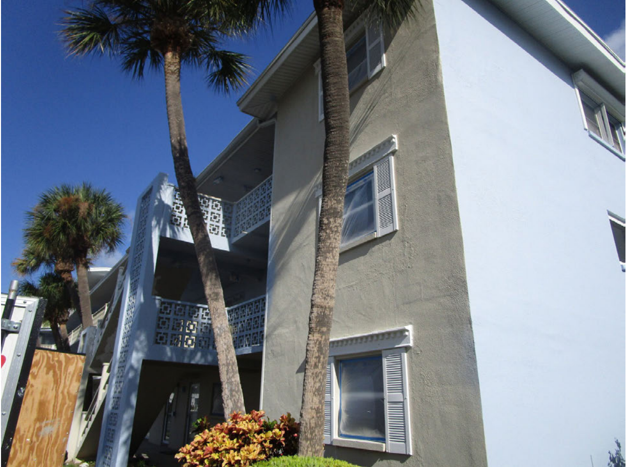
Exterior Elevation View. East Side. South Corner.
