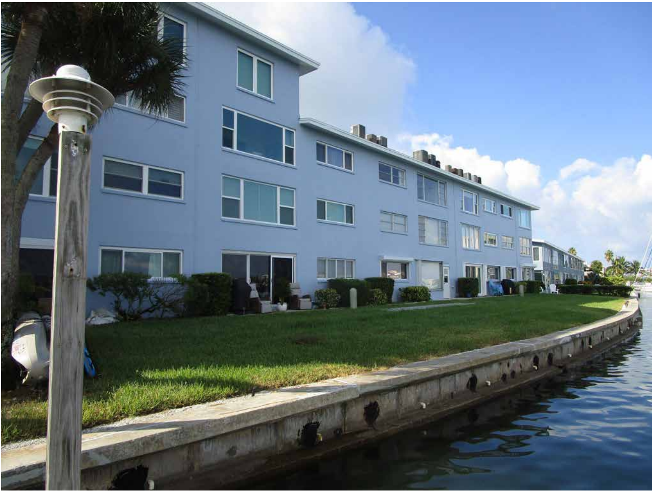
Capri Isle Garden Apartments No. 2. Exterior Elevation. North Side.
