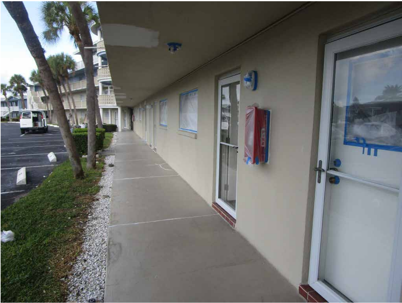
Capri Isle Garden Apartments No. 2. First floor hallway.
